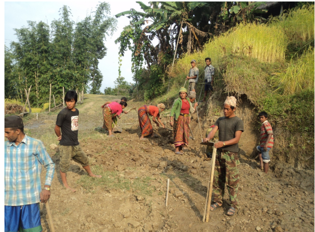
Group members engaged in construction works
