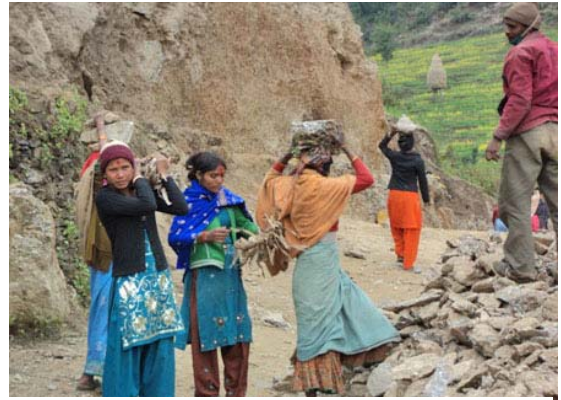
Kaushila carrying stones for constructing gabion wall
